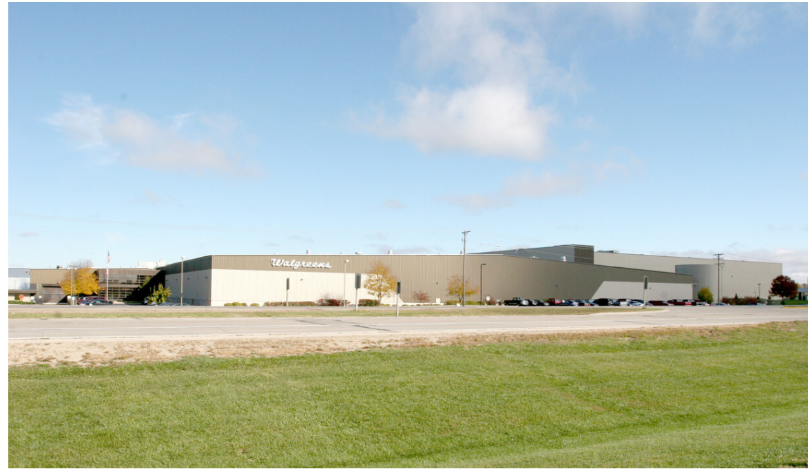
WALGREENS DC 4400 STATE HIGHWAY 19, WINDSOR
