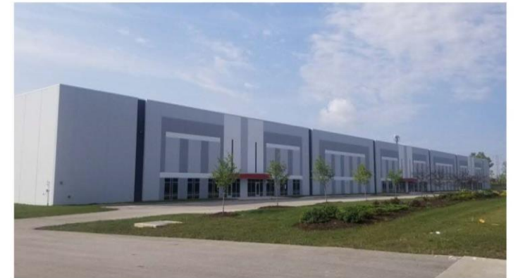
Spec industrial building at 12255 W. Carmen Ave., Milwaukee
