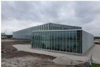
RICH KROHEN Contractors continue to work on Komatsu Mining Corp.'s new headquarters in Milwaukee's Harbor District on May 18, 2021. Komatsu Mining is on schedule with the complex.
